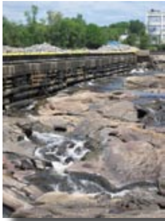
Timber crib portion of dam [west end]
