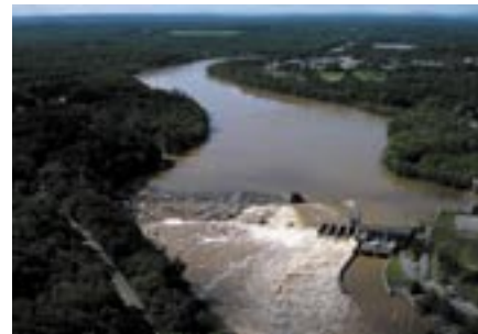
Worumbo looking upstream-coffer dam on left-post Hurricane Irene
