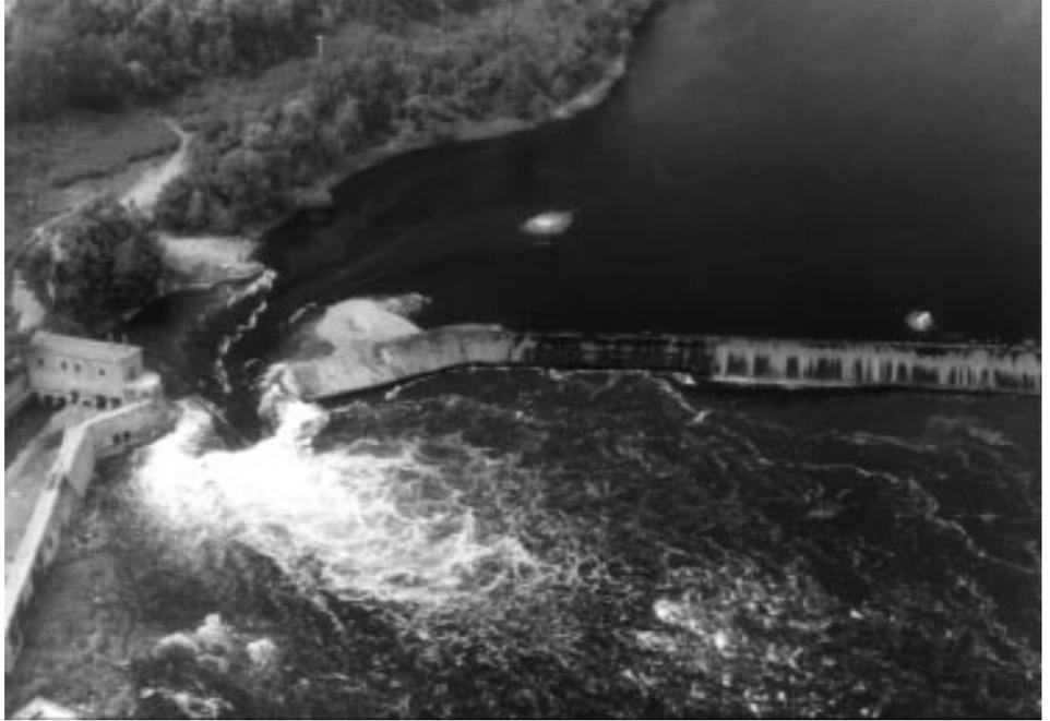
*July 1: A section of the coffer dam is removed by an excavator bucket christened with a bottle of champagne. The trickle of the Kennebec quickly increases to a torrent as it erodes the gravel dam and roars through the Edwards breach.*
