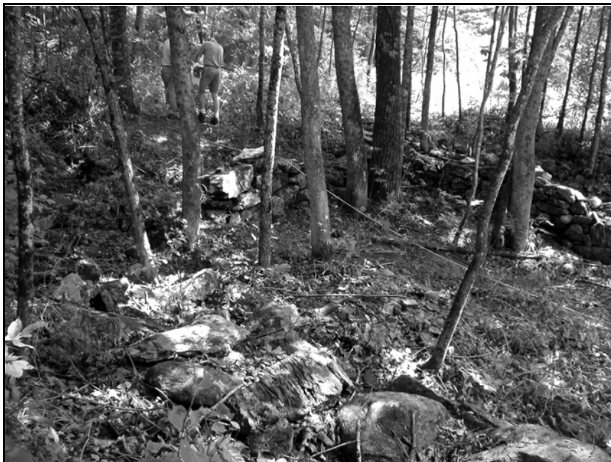
Figure 9. The inland (eastern) portion of the Carding Machine Mill foundation (away from the stream, which is out of the picture to the right).
