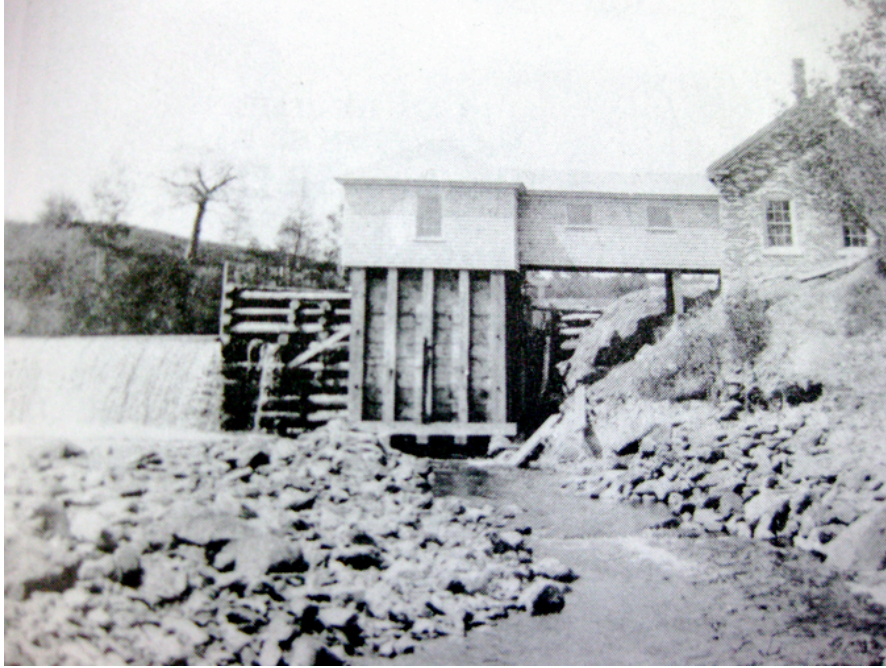
Figure 2.1. Dam and power house on St. George River circa early 1900s. From Whitten, 1990: 213. Courtesy, Edwin Boggs, Sr.
