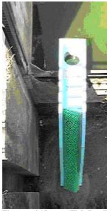
Figure 6.15. "Fish-Pass" prefabricated sluice-gate pass.
