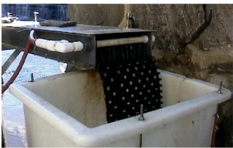
Figure 6.11. Akwadrain substrate extending beyond the top of the ramp at Greenville Dam eel pass. Photograph Alex Haro.
