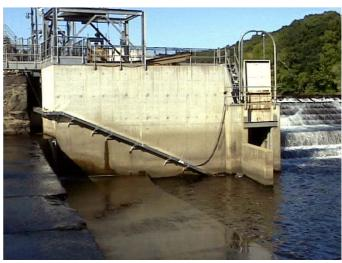
Figure 6.10. Eel pass-trap at Greenville Dam. Photograph Alex Haro
