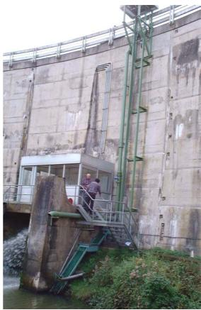
Figure 6.12. The Ville Hatte Dam eel lift. The substrate ramps can be seen below the platform.
