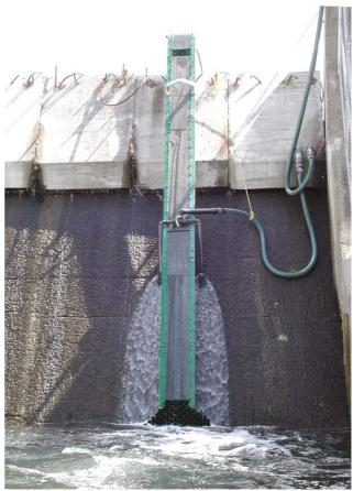
Figure 6.7. Eel pass at Chambly Dam. Note the breakwater blocks on the dam crest, and the gravity-fed attraction water being discharged from the two pipes part way down the dam face. Photo D. Desrochers.
