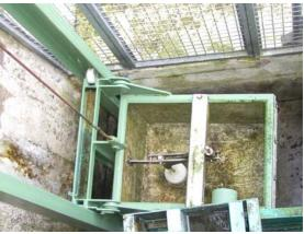
Figure 6.13. Lift hopper at Ville Hatte Dam eel lift in lower position.
