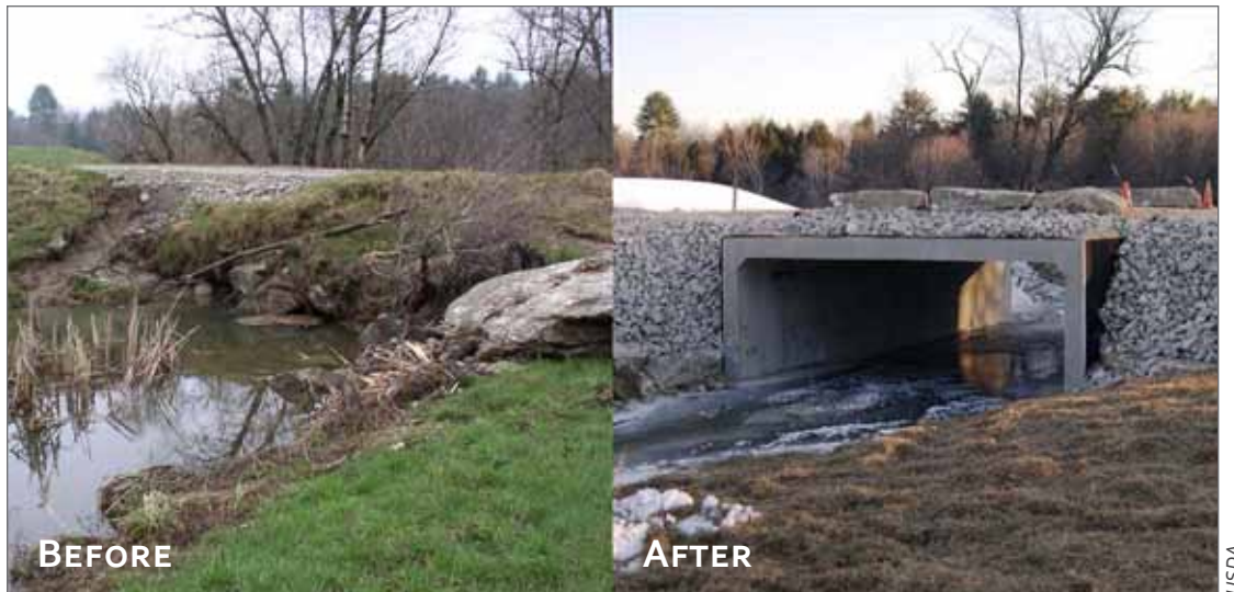
Left: Improperly installed culverts at road and rail crossings prevent fish from reaching their spawning and feeding areas, block the flow of nutrients, and cause other disruptions that harm ecosystem health. Right: Replacement with properly designed culverts helps fish to recover and can improve many aspects of ecosystem health. Thousands of culverts need replacing in Massachusetts, New Hampshire, and Maine.
