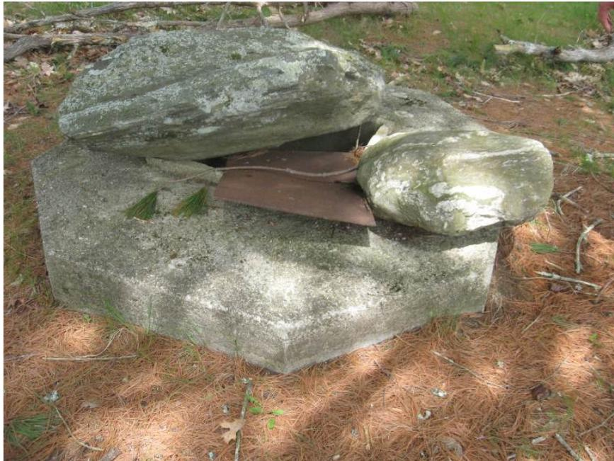
Haphazardly-placed stones and steel plate covering well near picnic shelter
