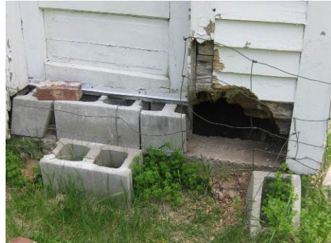
Structural Damage at Porcupine Entry into Gardiner-Dumaesque House
