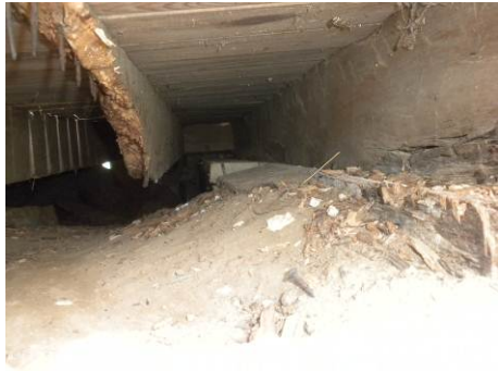
Structural Damage at Porcupine Entry into Gardiner-Dumaesque House
